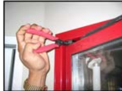
Disengage Hinge Pin
