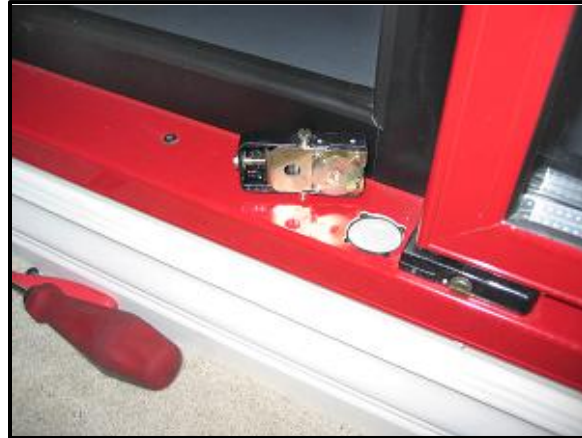
Mount Torquemaster
