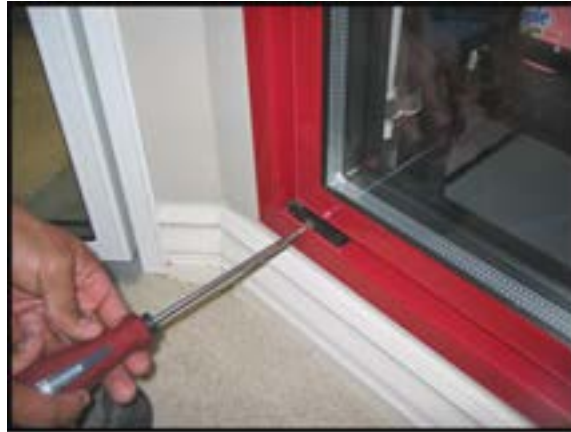
Release Torquemaster Tension
