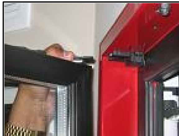
Withdraw from Hinge Gib
