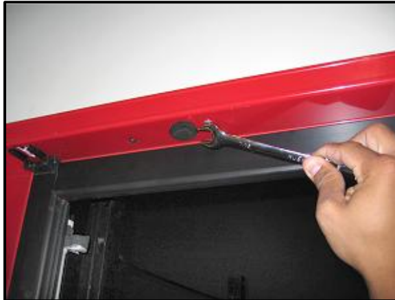
Tighten Hold-Open Bolt
