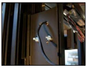
8. Place LED fixture over end mullion cover and drill one Ø 3/16" hole through slot of end cap on each end.
