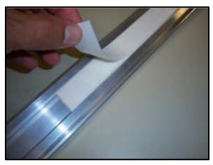
6. Cover exposed holes with foam tape supplied and feed wires through the tape and one of the upper holes.
