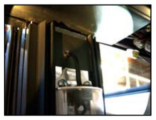
7. Attach LED fixtures to mullion using four #8-32 X 5/8" screws and nuts (supplied).
