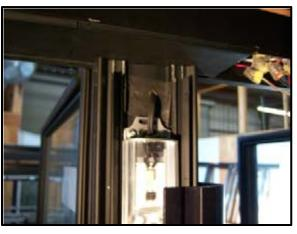
4. For the end mullion cover, carefully score plastic cover and snap extrusion section.
