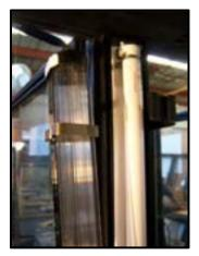
2. Detach mullion cover using a flat head screwdriver.
