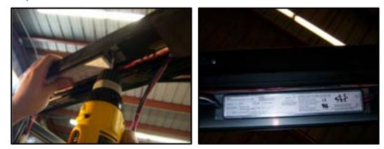
2. If no connector is found on driver, cut off blue and white wires from harness and connect to driver using Wago connectors or other Anthony approved connectors.
