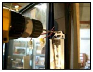
Attach LED fixture using #8-32 X 5/8" screws and nuts supplied. Proceed to wire fixture as described in step 6 of Installing LED Fixtures (Center Mullion) Model 401.
