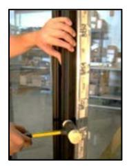
Note: Seal any open holes using neutral cure silicone to prevent air infiltration.
