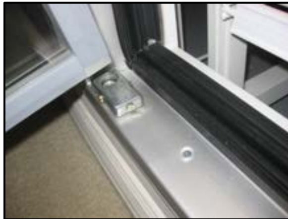
Insert Torque Rod into Torquemaster
