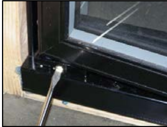
Release Torquemaster Tension
