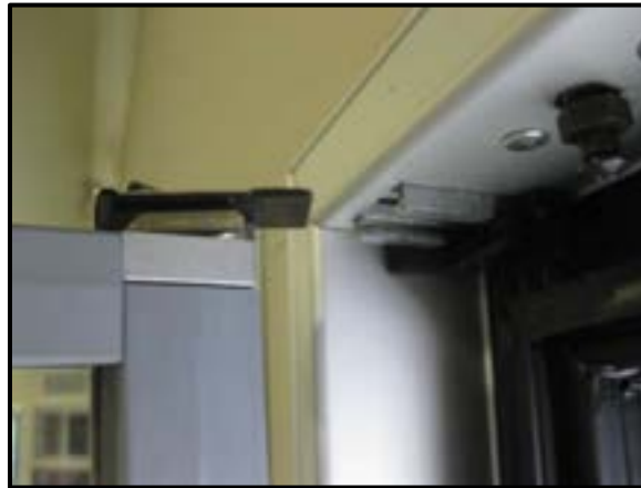
Withdraw Away from Hinge Gib
