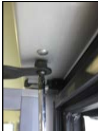
Remove Hold-Open Bolt
