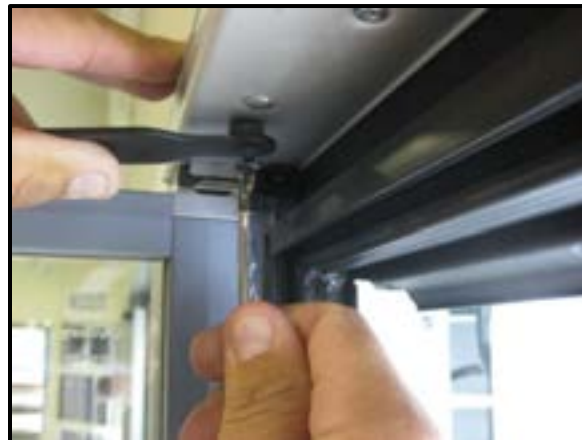
Tighten Hold-Open Bolt
