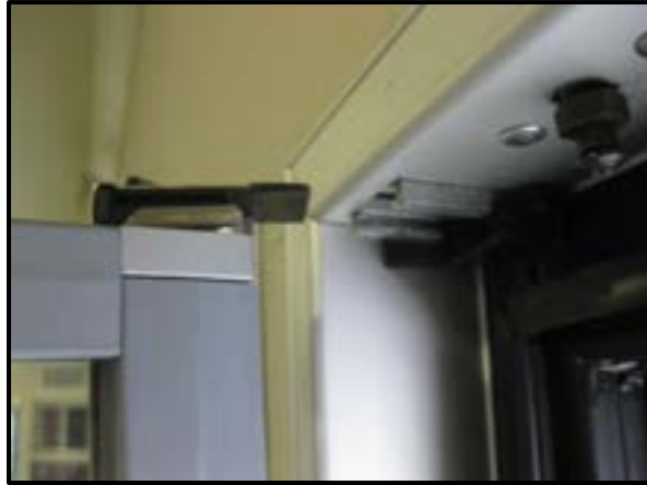
Connect Hinge Pin
