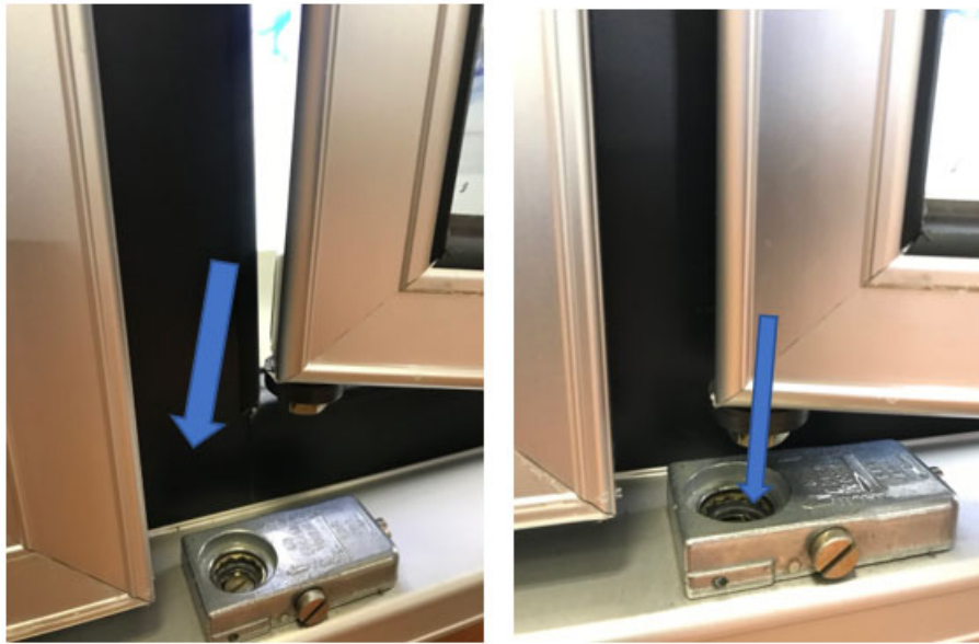
Figure 4.1: Seating Door onto Torque Master
