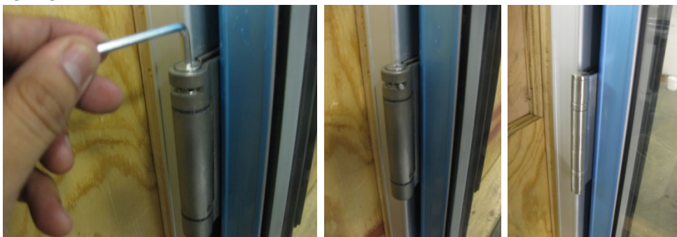
Figure 18.16: Torquing Hinges
