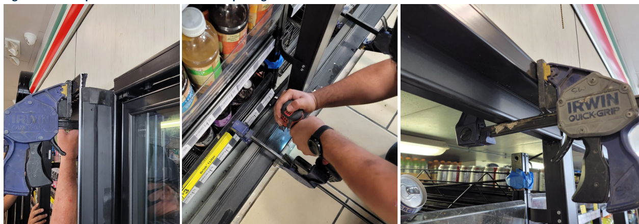
Figure 2.2: Clamps to insert Frame into Net Opening
