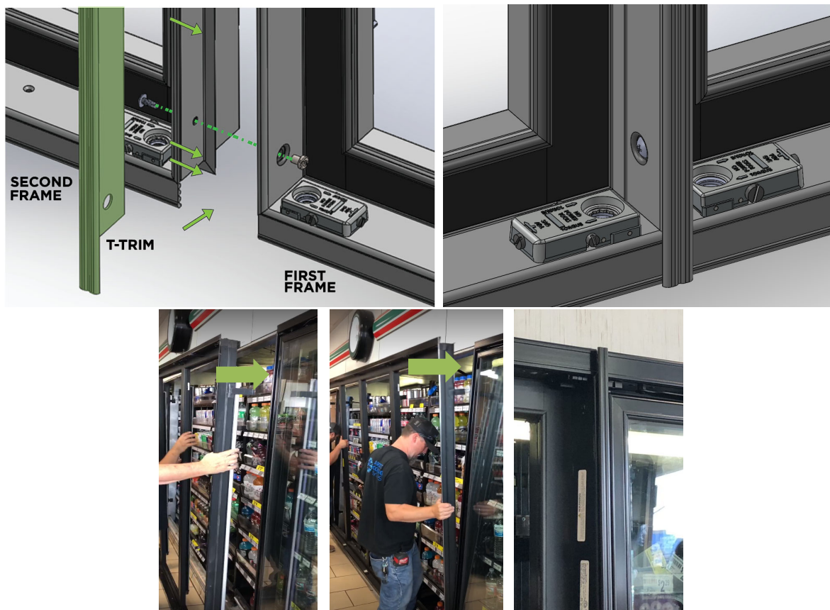
Figure 2.6: T-Trim installation
