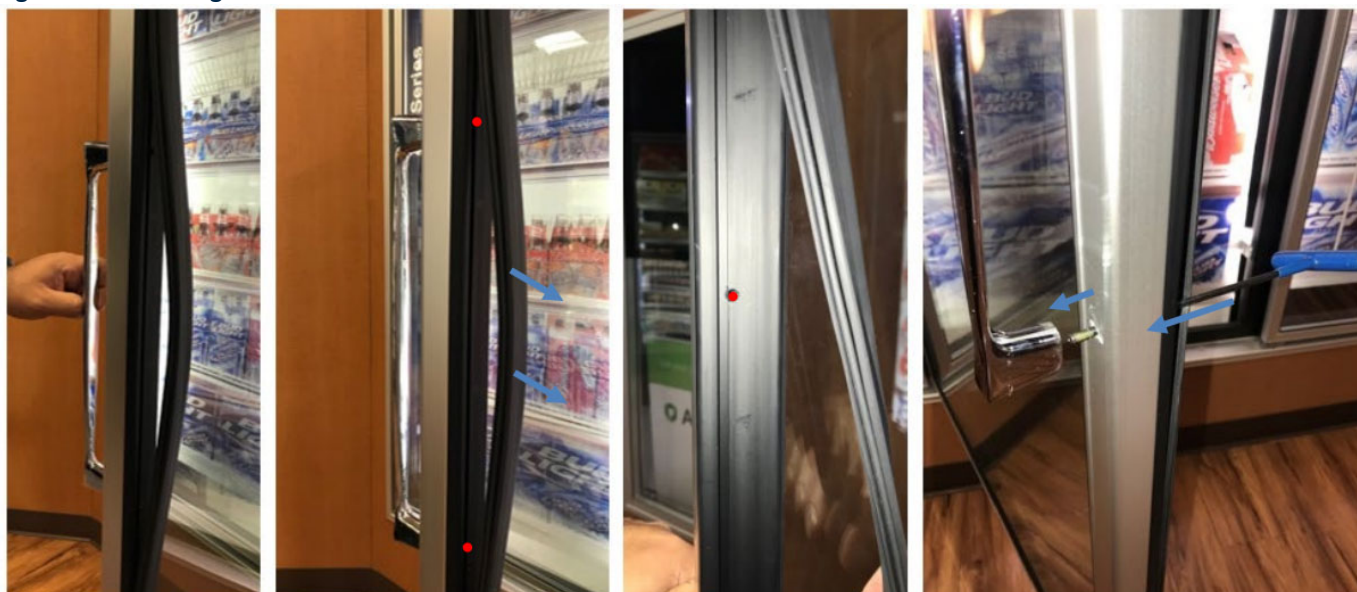
Figure F.1 – Locating handle screws
