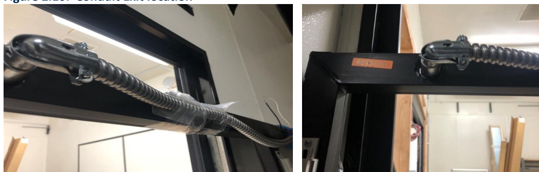
Figure 2.10: Conduit Exit location
