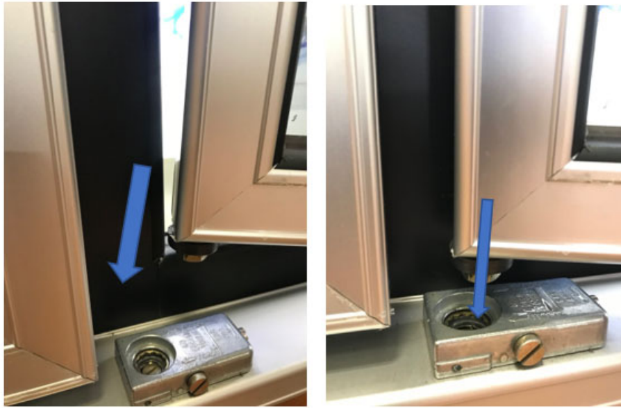
Figure 4.1: Seating Door onto Torque Master
