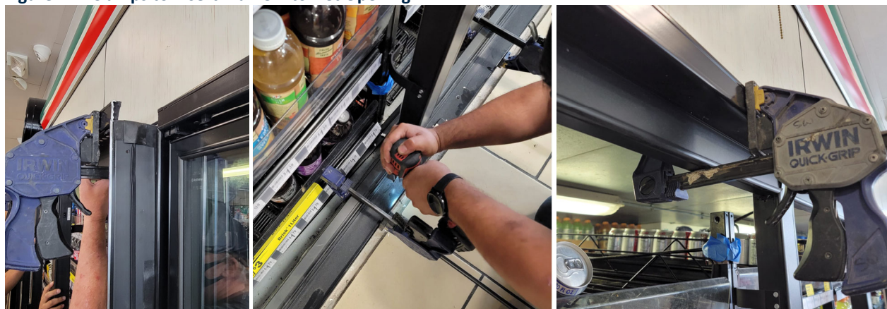
Figure 2.2: Clamps to insert Frame into Net Opening
