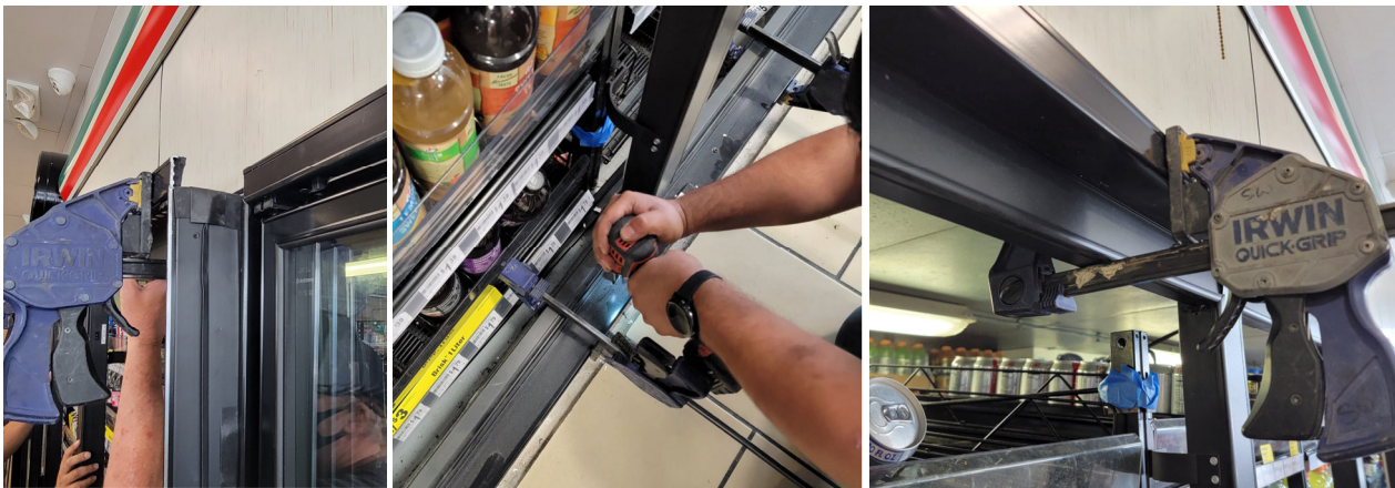
Figure 2.2: Clamps to insert Frame into Net Opening
