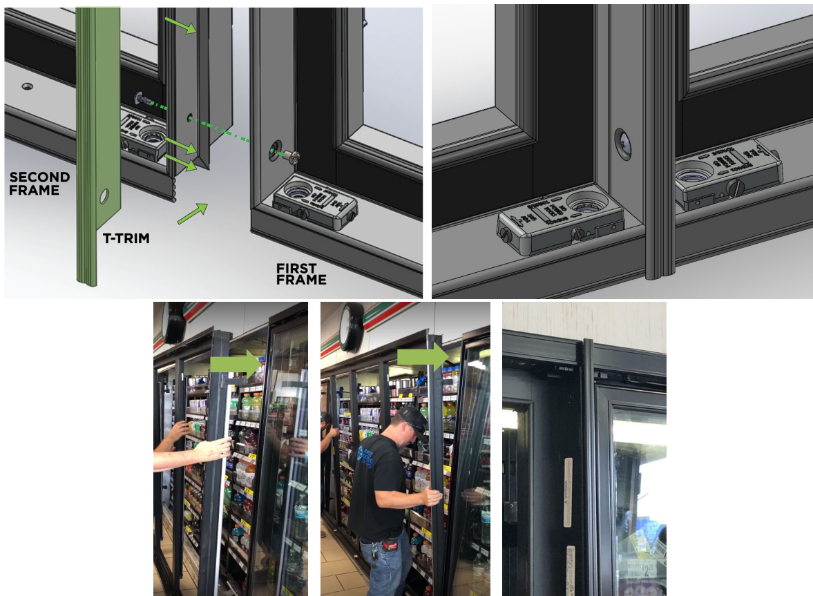
Figure 2.6: T-Trim installation
