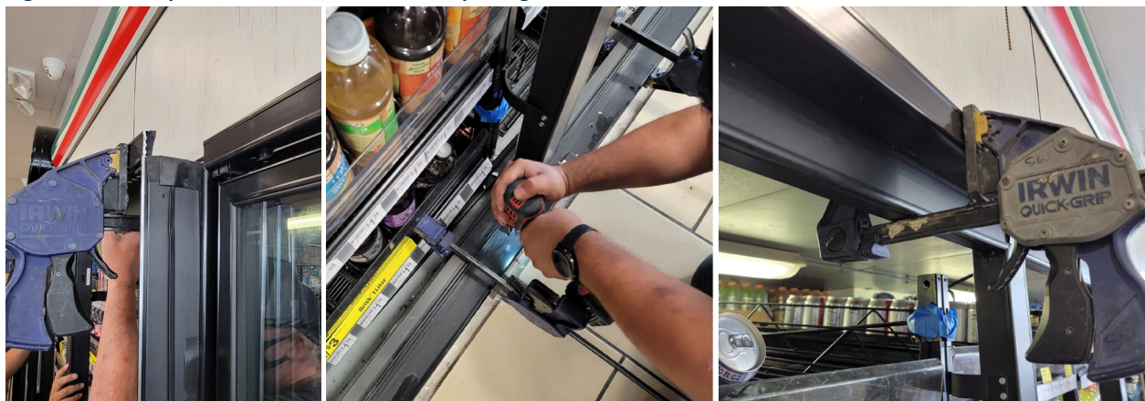
Figure 2.2: Clamps to insert Frame into Net Opening
