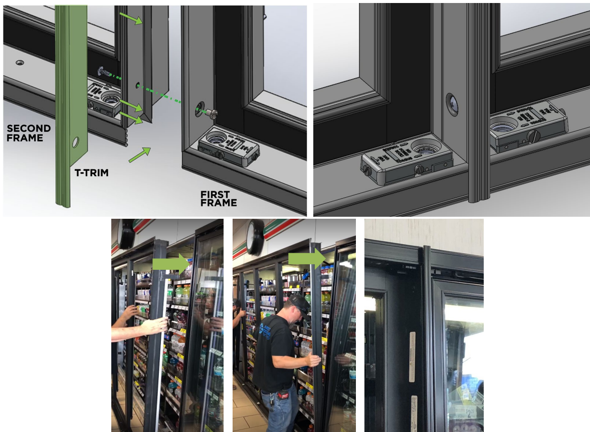
Figure 2.6: T-Trim installation
