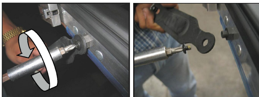
Figure 14.1 Removing hold-open assembly from door.
