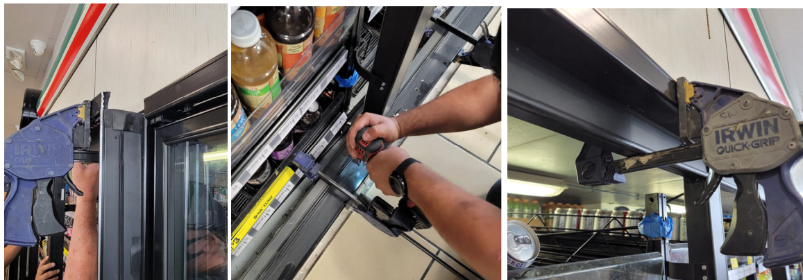
Figure 2.2: Clamps to insert Frame into Net Opening
