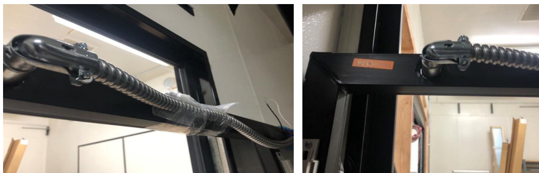
Figure 2.11: Conduit Exit location
