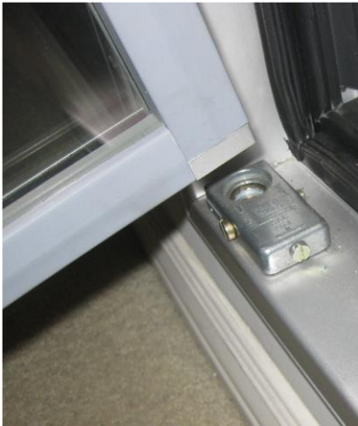
Figure 7 Insert Torque Rod into TorqueMaster
