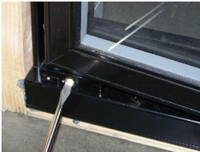
Figure 10 Release TorqueMaster Tension
