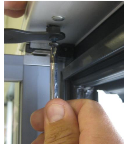
Figure 9 Tighten Hold-Open Bolt
