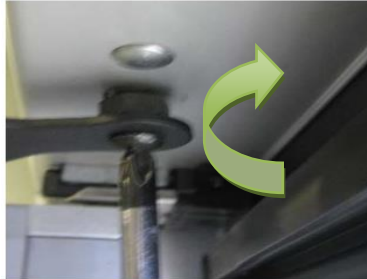
Tighten Hold-Open Screw
