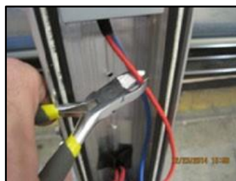
Cut wires at the bottom of the driver (red & blue)
