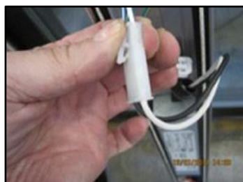
Disconnect wire connector at top of driver (black & white)
