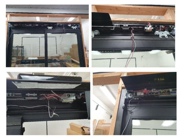
Connect external power to the black and white wires identified as " external power 120V ", outgoing from Anthony AEC. Route wires carefully, without affecting the operation of moving parts.
