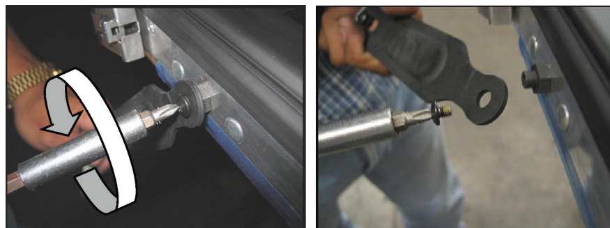
Figure 13.1 Removing hold-open assembly from door.
