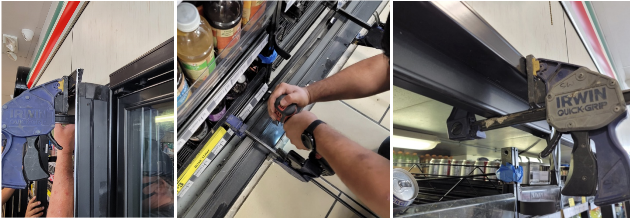
Figure 2.2: Clamps to insert Frame into Net Opening
