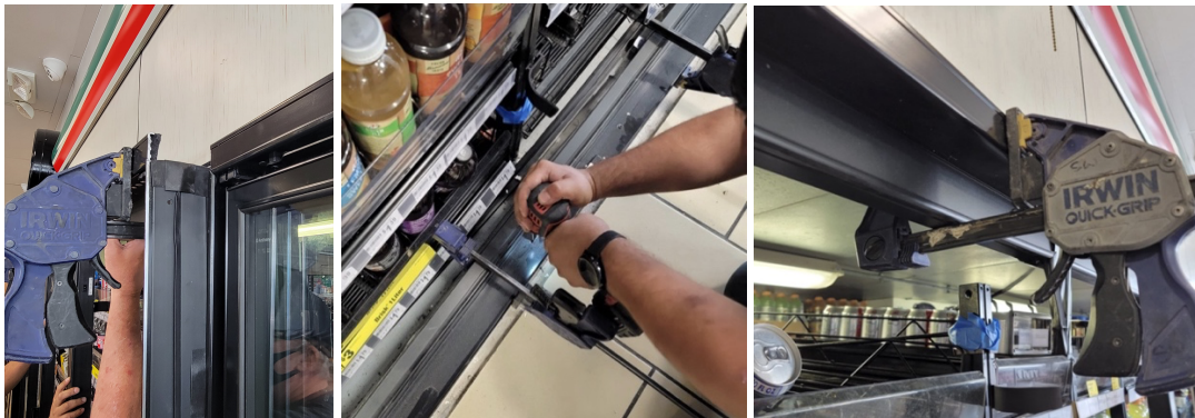
Figure 2.2: Clamps to insert Frame into Net Opening
