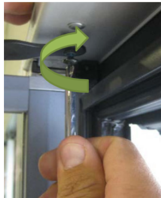
Figure 7.1: Secure hold-open mounting screw.
