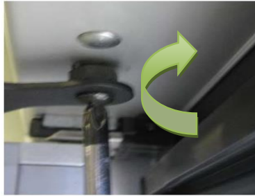
Tighten Hold-Open Screw
