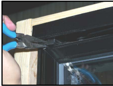
Disengage Hinge Pin
