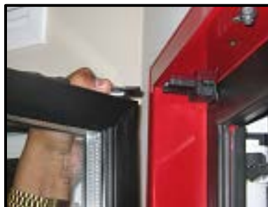
Connect Hinge Pin
