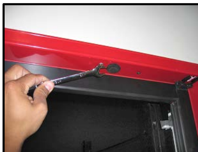
Remove Hold-Open Bolt
