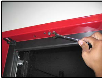
Tighten Hold-Open Bolt
