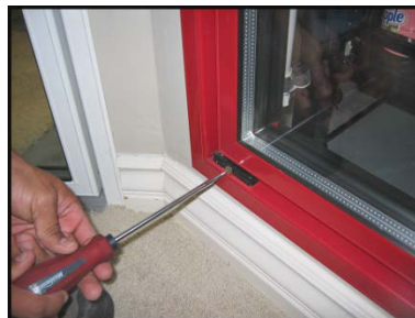
Release TorqueMaster Tension
