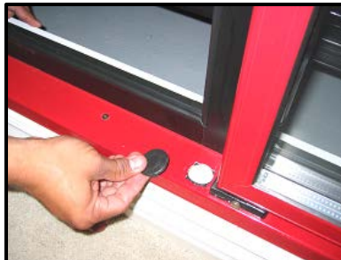
Remove Plug Gap
