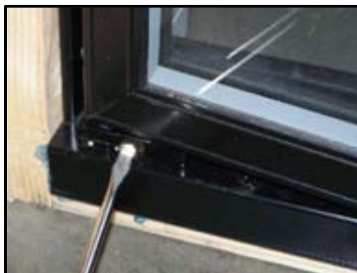
Release TorqueMaster Tension
