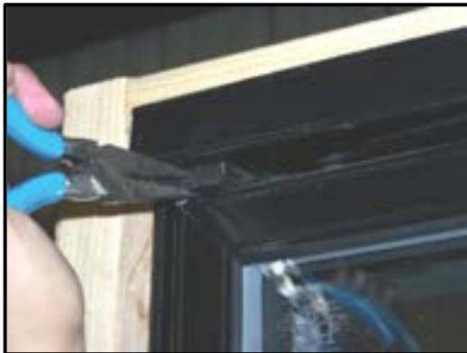
Disengage Hinge Pin
