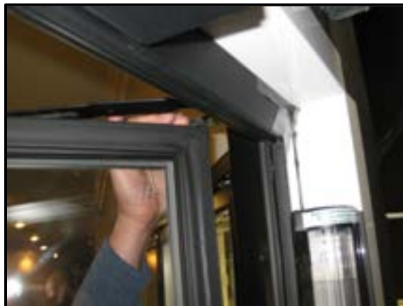
Withdraw Away From Hinge Gib
