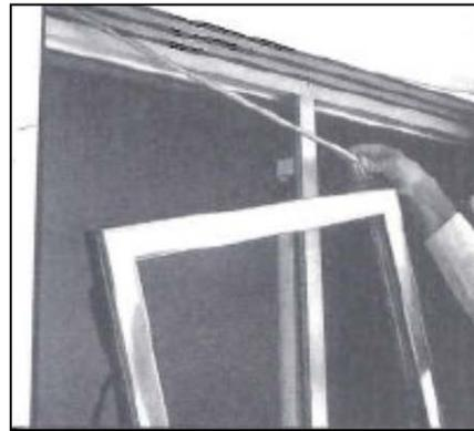
4. With spring attached, lift door into top rear track.
