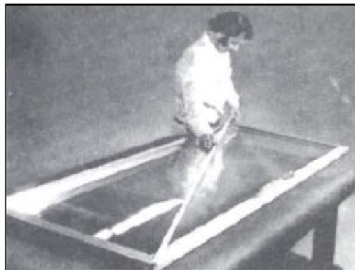
8. After the glass unit has been replaced and door rails are in square, re-insert heater wires in door rail and replace the retaining strips.
