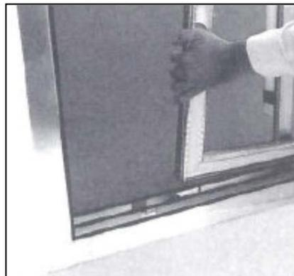
6. ***Note that Roller cage does not screw into bottom of door.***
