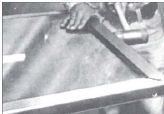
7. After door has been re-built, measure door diagonally to check for square.
