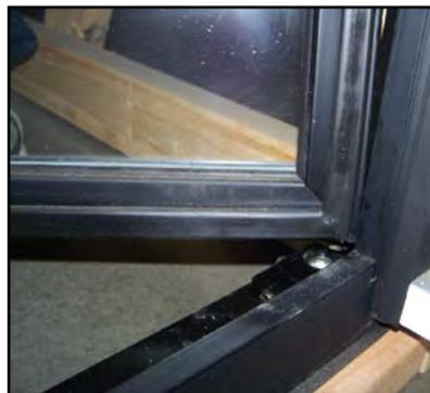
3. Engage the door with the hinge pin plug inserted into hinge pin plug receptacle at top of frame.
