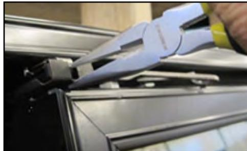
4. Lift door out of Torquemaster. Lean door on its side against a stable surface.
