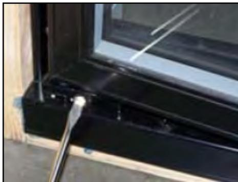
8. Do not use power tools for installation or removal.
