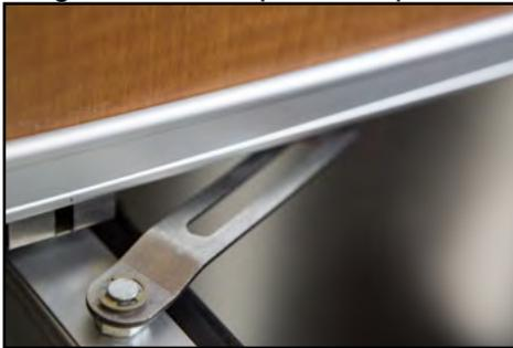
6. Adjust the closing force by turning the screw on the front of the Torquemaster with a flat-head screwdriver. Turn counter-clockwise to tighten, clockwise to loosen. **Over-adjustment will cause door to slam.**
