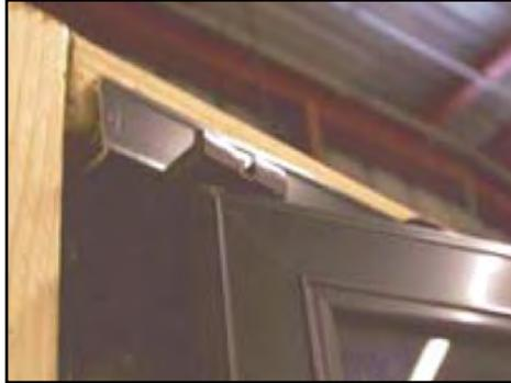
4. Push the door into the top of the frame with your thumb until the hinge pin plug snaps into place.
