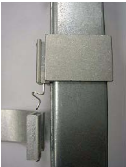
Figure 1 Align brackets
