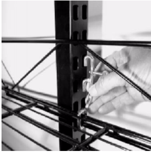
Figure 11 Insert S-hook onto post
