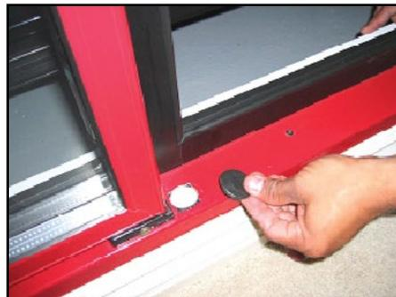
4. Place the Torquemaster on the newly opened mounting pocket in the frame, with the hollowed end of the Torquemaster towards the frame.
