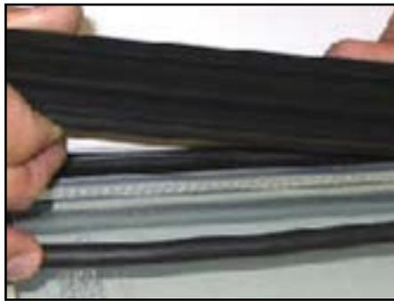
10. Check the entire plastic cover and confirm that both the inside and outside lips are fully inserted into the door rail grooves.
