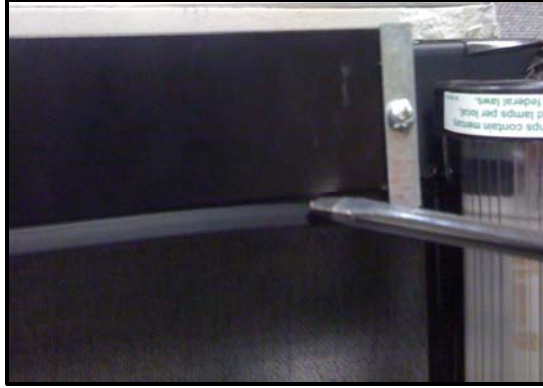
Raceway Cover Slip Removal
