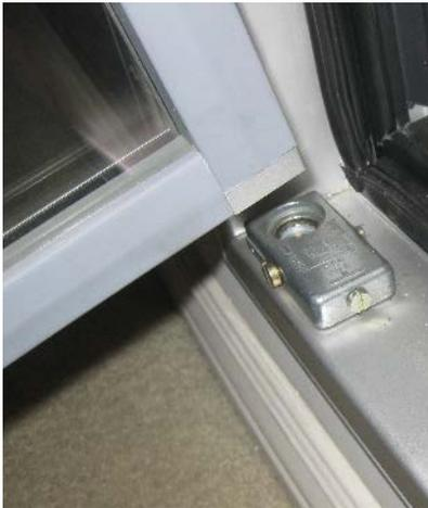
Figure 7 Insert Torque Rod into TorqueMaster
