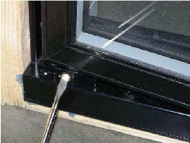
**Figure 10 Release TorqueMaster Tension**
