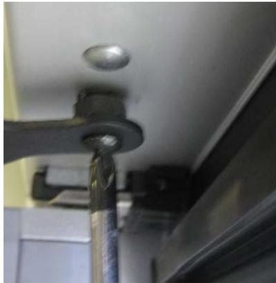
**Figure 11 Remove Hold-Open Bolt**
