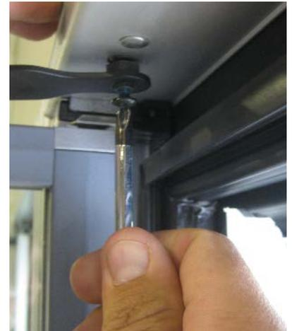
Figure 9 Tighten Hold-Open Bolt
